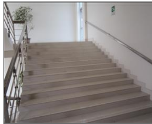
Photo of the inside of the main production hall Facility staircase.JPG
