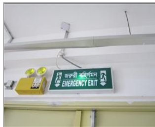
Photo of the inside of the main production hall Emergency exit sign.JPG
